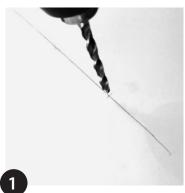
Check product orientation. Mark hole positions from brackets pre installed on MOMO base (2 per metre/40") and drill if required.
